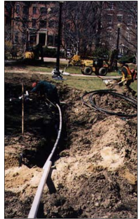
Installing the irrigation system, Public Garden
